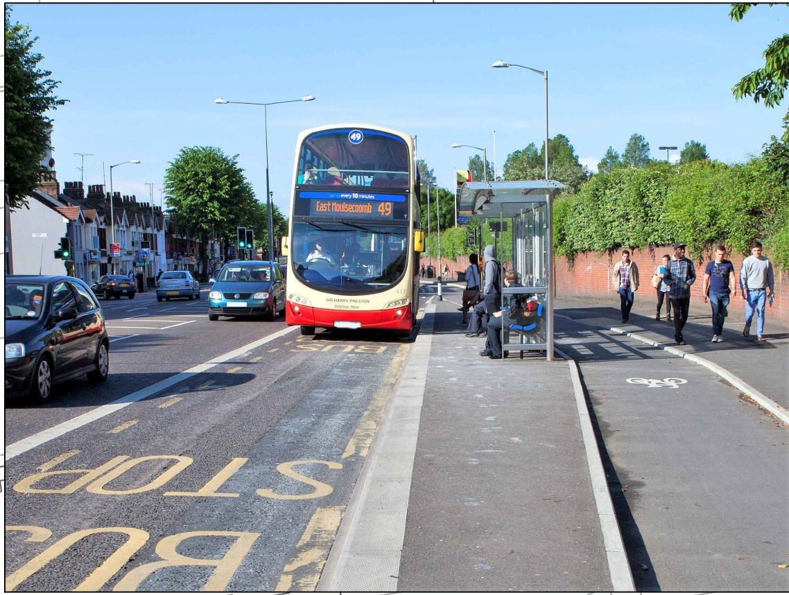
Image 2 - Example of floating bus stop
