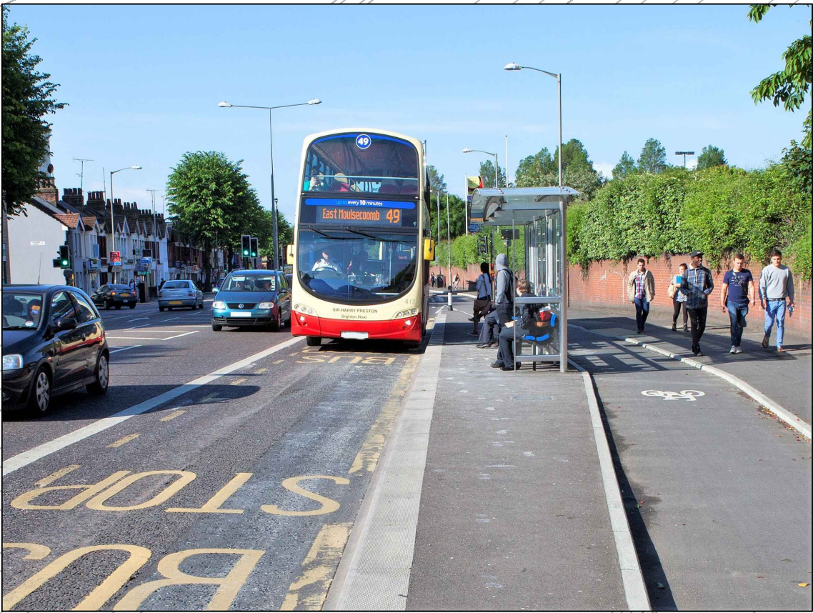
Image 2 - Example of floating bus stop
