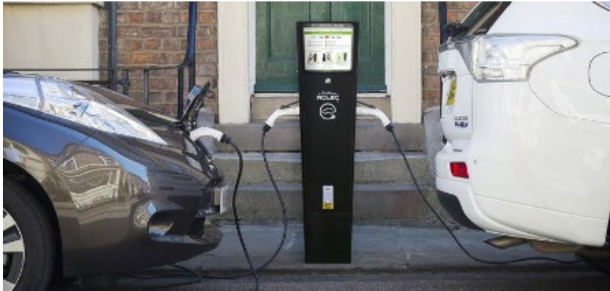
An example of on street charge point. (picture from Zapmap)
